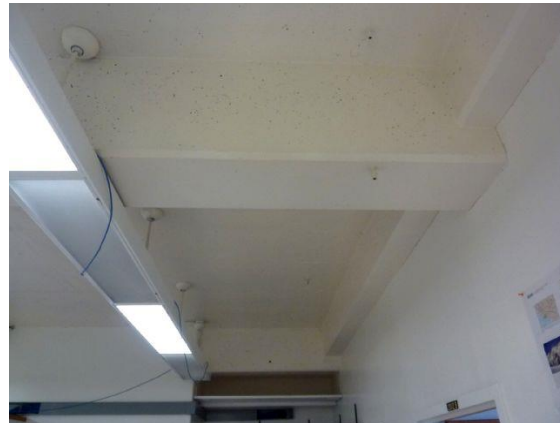
Level 2 Overhead Exposed Ceiling Area
