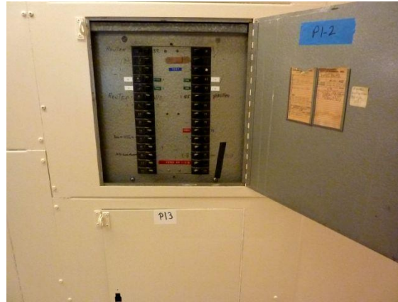
Level 1 Typical Electrical Panelboard Branch Circuits
