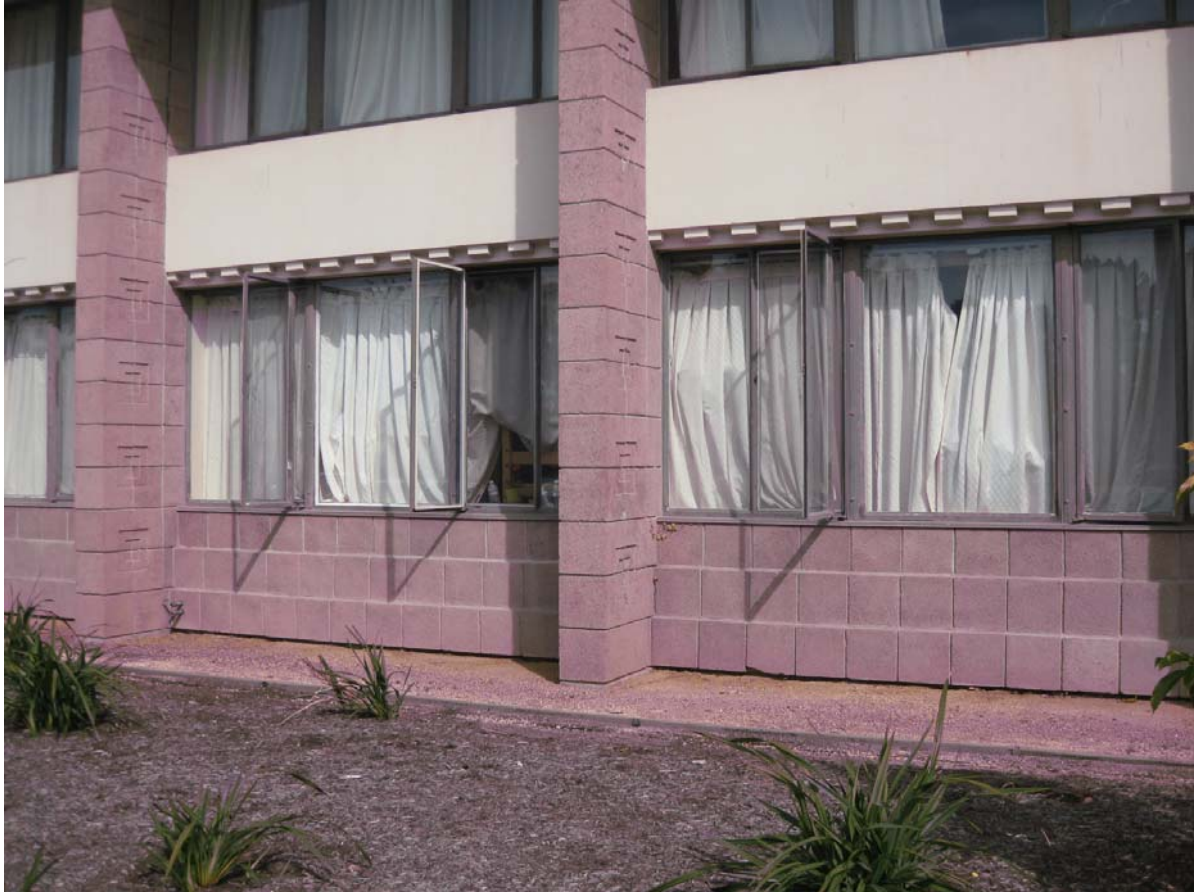
Typical Exterior Windows
