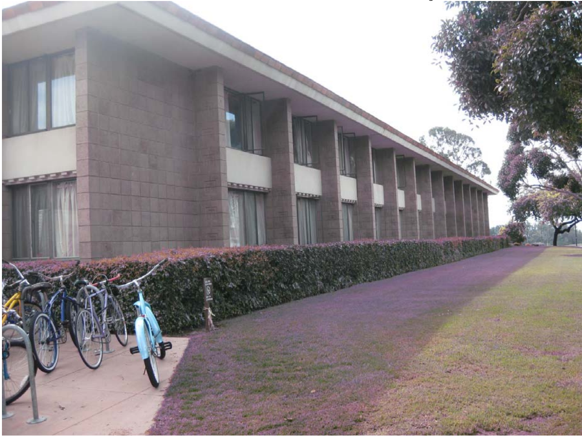
West Exterior (Partial)
